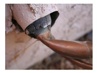
Just like blowing across the top of a soda bottle, refrigerant flow through a line set can generate a whistle affect. Whistle noises can be found in any part of a system or line set; but they are typically found in areas of high velocity such as discharge lines.
