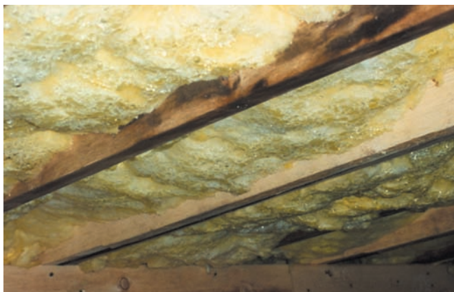
Photo 1 (left): Icky crawlspace. Note the condensation on the underside of the fiberglass batt insulation and the rot at the exposed portions of the crawlspace floor joists. Photo 2 (right): Ventilation opening. Crawlspace has plenty of cross ventilation and good drainage.
