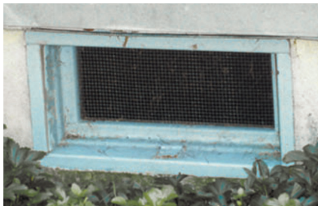
Photo 1 (left): Icky crawlspace. Note the condensation on the underside of the fiberglass batt insulation and the rot at the exposed portions of the crawlspace floor joists. Photo 2 (right): Ventilation opening. Crawlspace has plenty of cross ventilation and good drainage.
