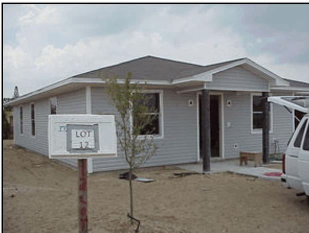
Figure 20. Sealed attic home under construction in Ft. Myers, FL. Conventional dark gray shingles were used.
