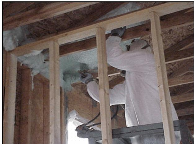
Figure 21. Insulating foam being applied to a 5-inch depth on the under side of the roof.
